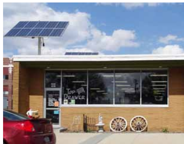
Figure 33: A recent past building is modified with solar panels to enhance its energy efficiency.
