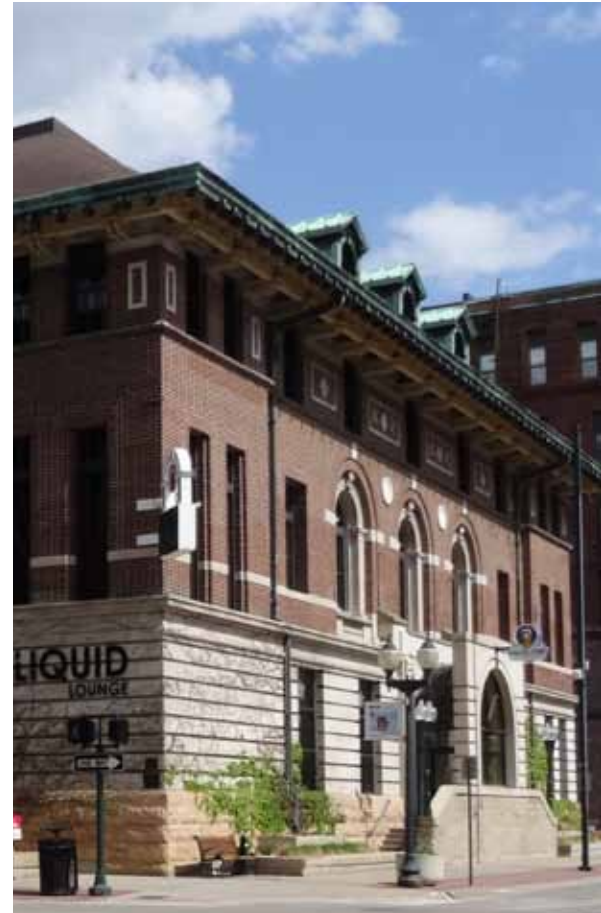
Figure 8: Heritage tourism is another benefit of investing in historic preservation, as people are attracted to the cultural heritage sites within an area. These resources provide visitors a link to Cedar Rapids' history and an understanding of its contribution to state and national history.
