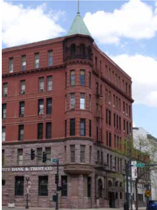
Figure 92: Cedar Rapids Savings Bank (Guaranty Bank) (1895-1909) at 302 Third Avenue SE. Designed by Cedar Rapids architects Henry Josselyn and Eugene Taylor.
