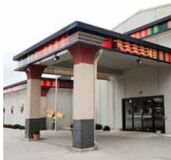
Figure 64: African American Museum of Iowa at 55 12th Avenue SE. Source: Web
