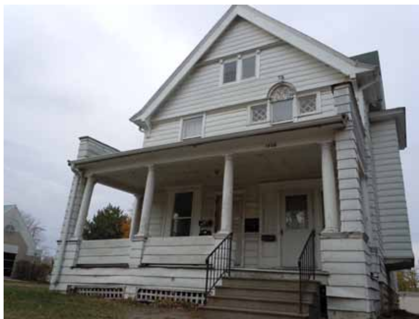
Figure 54: 1300 Third Avenue SE. Source: Web
